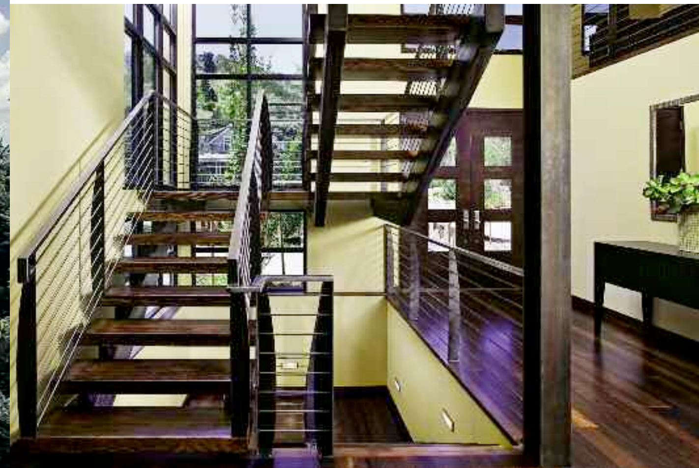
ON THE RISE The open risers of the stairwell to all three floors allow the view and light to show through to the interior.
